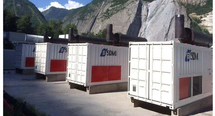
*Pic. 2. The four 1900 kVA generating sets installed at the foot of the Pas-du-Roc cliff*
