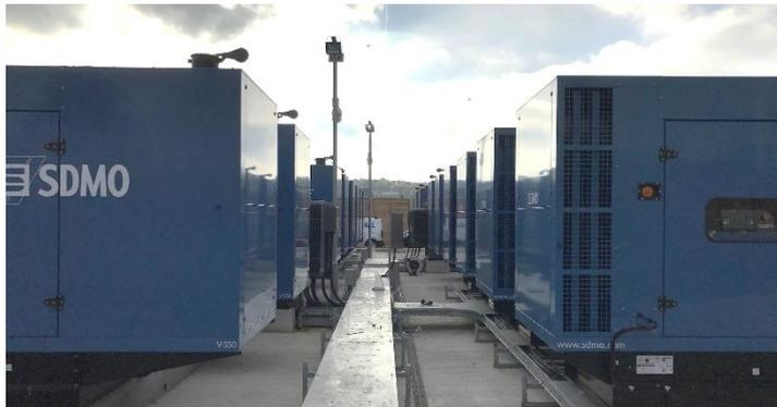
The generating sets supplied are perfectly suited to this requirement as they provide output of 400 kW LTP (Limited-Time running Power). This means that they are able to provide 100% of their power at constant load for 500 hours each year.
