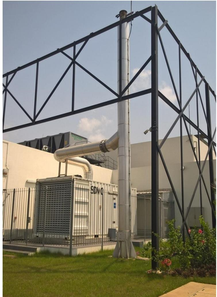
*Photo 3: One of the two 1400 kVA generating sets installed near the data center.*
