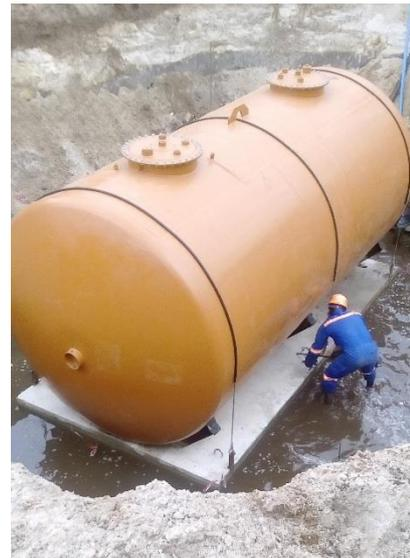
*Photo 2: One of the two 25,000-liter tanks being installed on the site*
