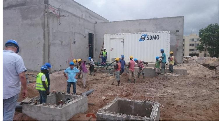
*Photo 1: On-site installation of the two 1400 kVA generating sets*
