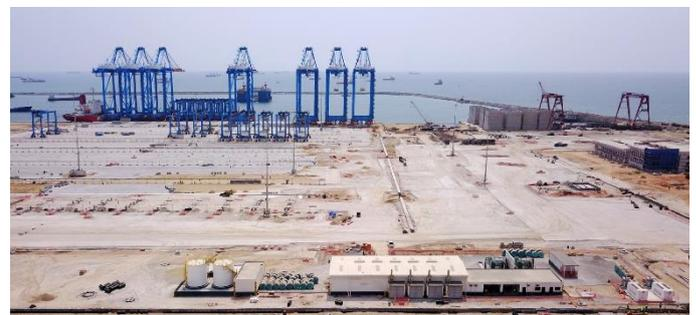
*View of the outside of the backup power plant in the foreground with two fuel tanks (left), and the building housing the four generating sets (center)*
