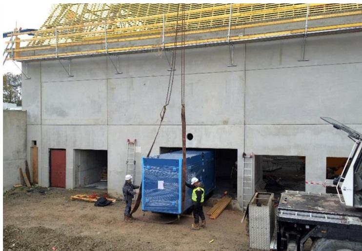
*Pic. 2: Installation of the 550 kVA generating set in the specially constructed 27m<sup>2</sup> equipment room*
